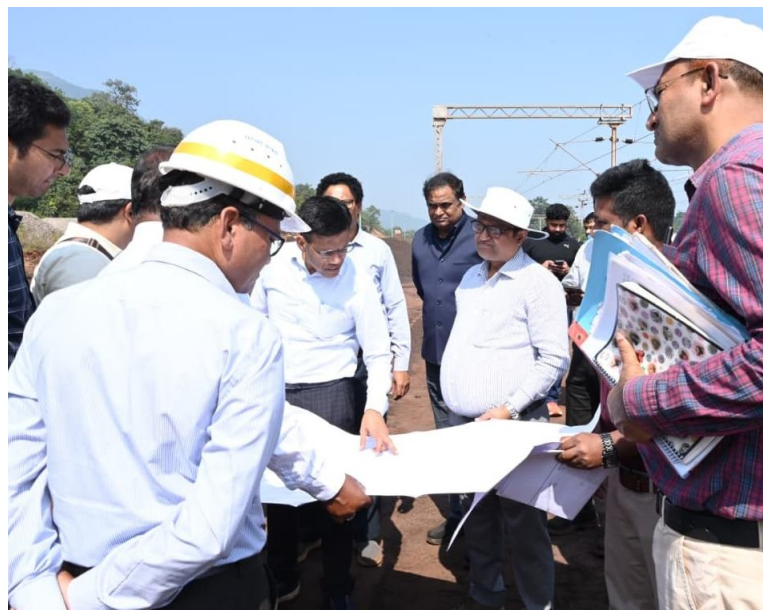
DRM Shri Lalit Bohra inspection of the NMDC sidings and loading points at Kirandul and Bachel
